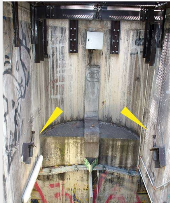
A heavy, five-ton barrier safely stopped by MAGNUM shock absorbers J.P. van Eesteren B.V., 1006 BD Amsterdam, Netherlands
